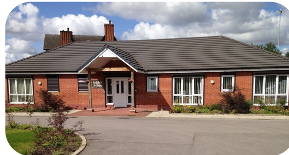
Talbot House Support Centre building
